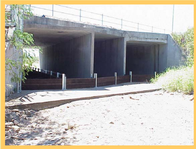
View from upstream - nib walls in place
